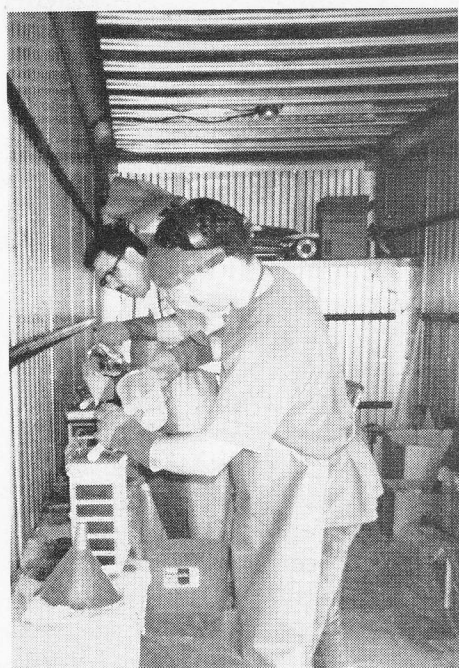
B.A.T.'s team fills the cells with sodium hydroxide (NaOH) electrolyte.
